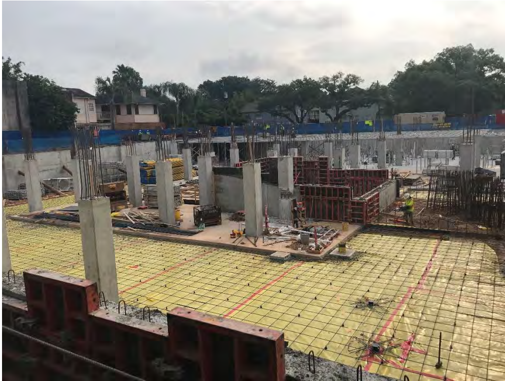
4/21/20- View northeast from western side, basement parking entry ramp being formed, vapor barrier installation, columns poured to grade
