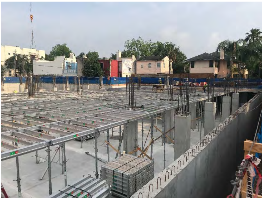
4/21/20- View northwest from eastern side, basement parking slab partially poured, post tension slab being formed at grade
