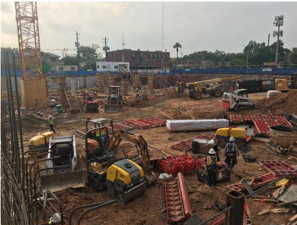
4/21/20- View southeast from western side, form work lay-down area, temporary entry drive, construction trailer
