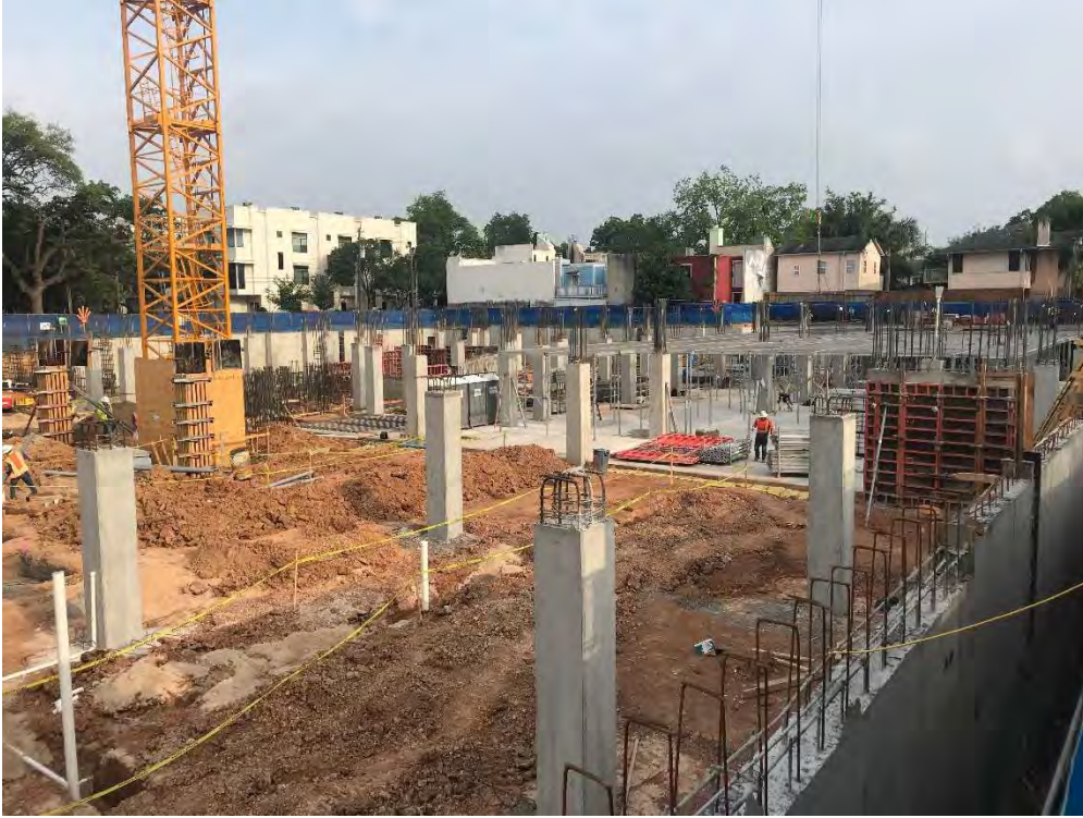
4/21/20- View northwest from southeastern corner, underground plumbing being roughed in, columns poured to grade, tower crane installed
