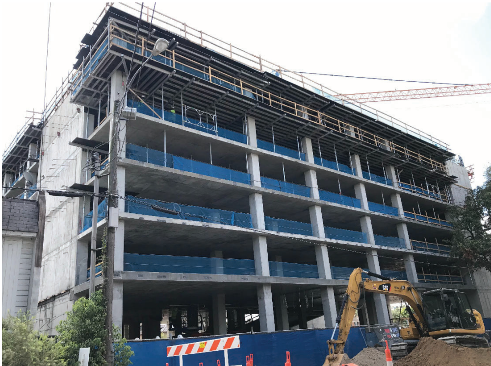
7/11/20- View southeast from Grant Street, last garage post-tension slab formed, shoring installed, embed plates installed for decorative garage screening, storm sewer connection backfill in process
