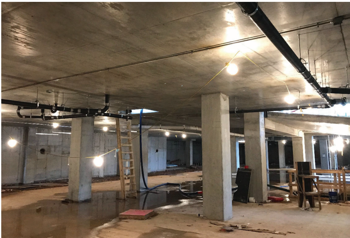
6/25/20- View of northern basement wall, plumbing and electrical beginning rough-ins, temporary lighting installed
