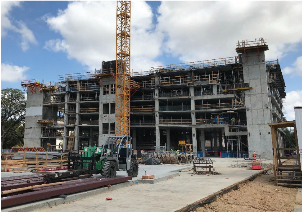
7/11/20- View northwest from southeastern site corner, last garage post-tension slab formed, shoring installed, level one post-tension slab poured
