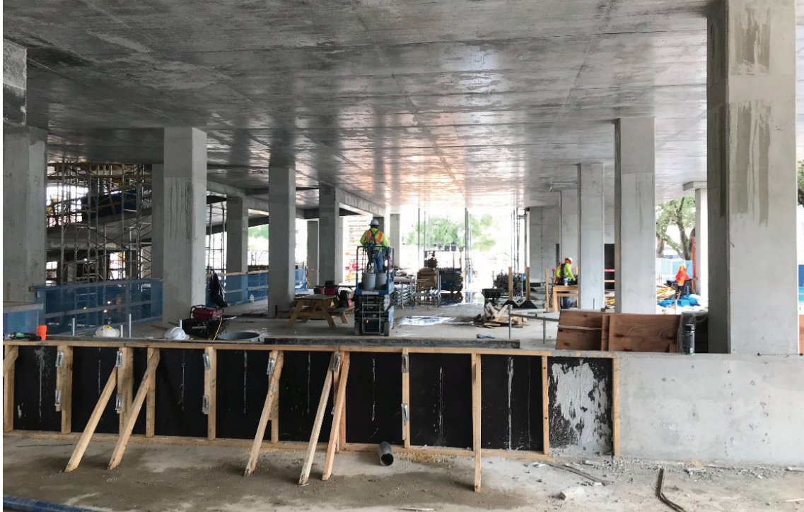
6/25/20- View south from northwestern portion of first floor garage, concrete barrier wall being formed, concrete column touch-up in progress
