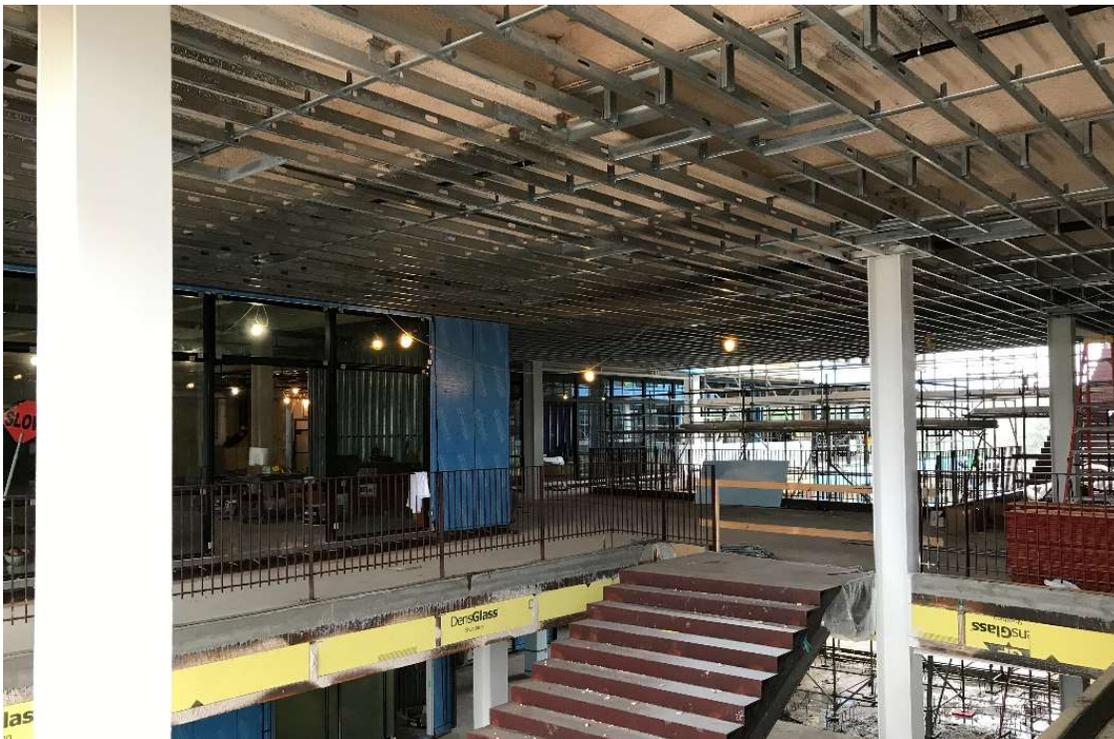
2/10/21- Level 2 soffit being framed, intumescent columns being finished
