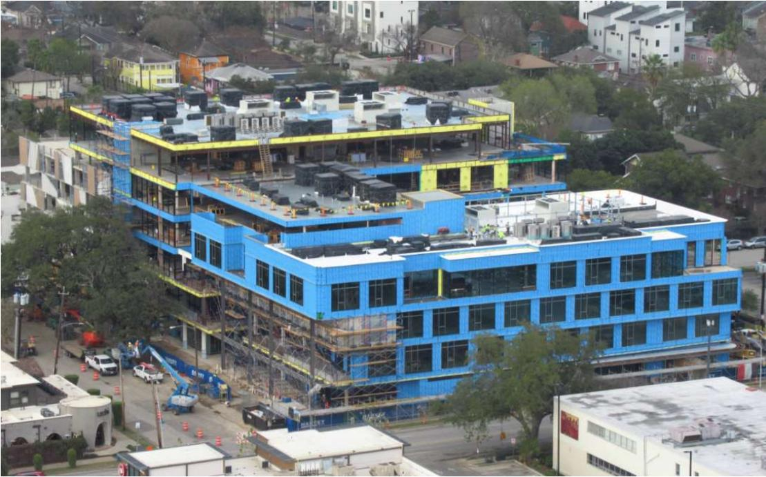
2/9/21- Aerial view northeast, level 3 brick installation underway, majority of glazing installed on levels 3 and 4
