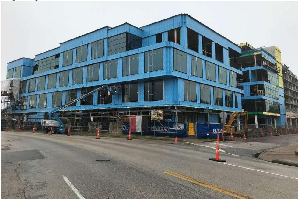
2/10/21- View northwest from southside of Westheimer, level 3 brick installation underway, majority of glazing installed on levels 3 and 4
