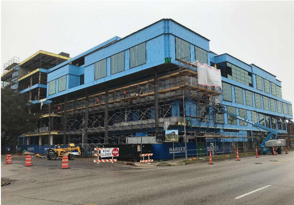
2/10/21- View northeast from southside of Westheimer, level 3 brick installation underway, majority of glazing installed on levels 3 and 4
