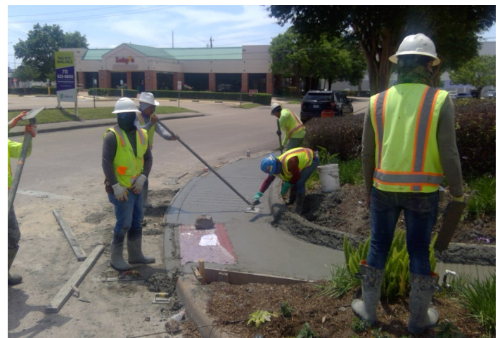
Finishing Ped Ramp and Installing Truncated Domes Mat.
