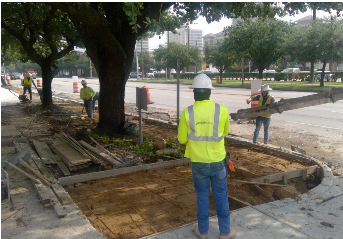
Form work for sidewalk installation
