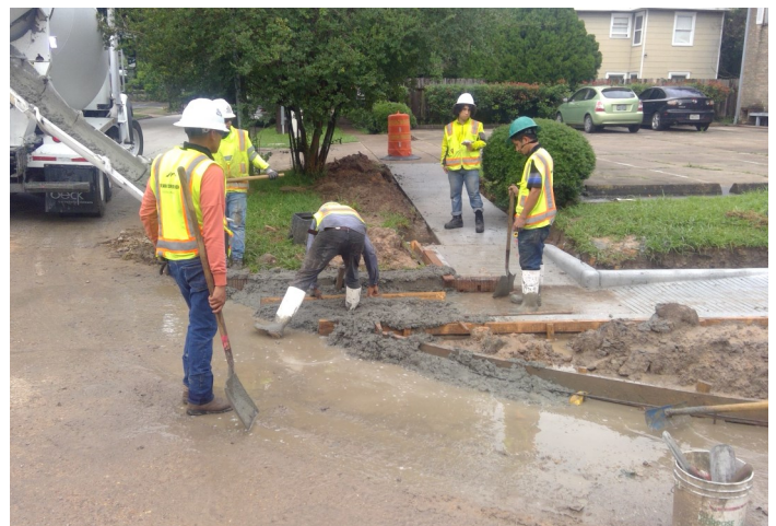
Curb ramp Installation
