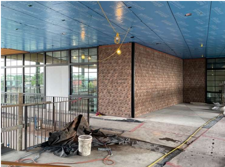
6/9/21- Second floor terracotta shingles installed
