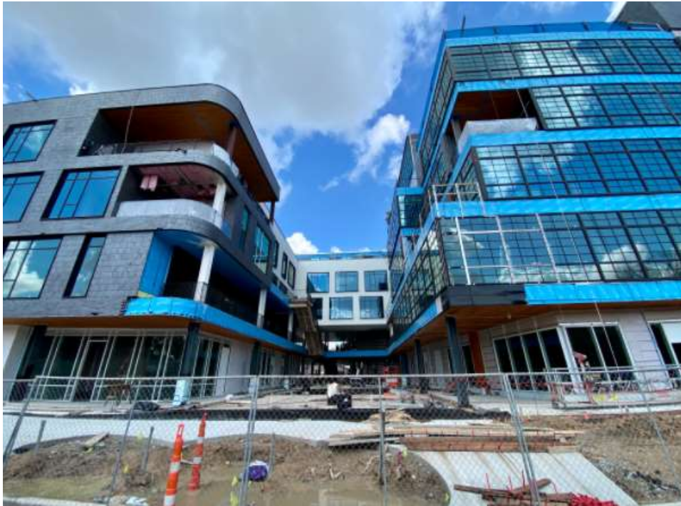
6/5/21- view of paseo, metal panel mock up in place, sitework concrete poured
