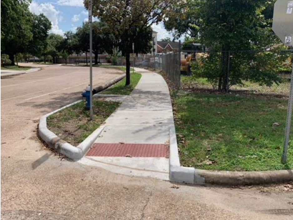
After Construction – Intersection of Haddon St and Commonwealth St
