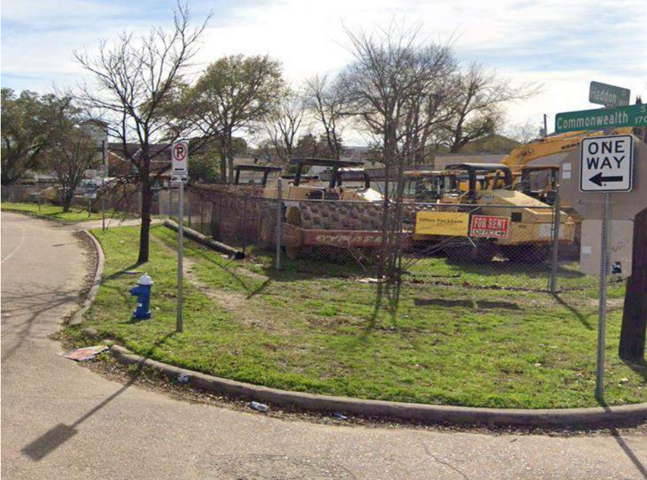
Before Construction – Intersection of Haddon St and Commonwealth St
