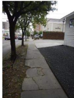
Back of Curb Condition
