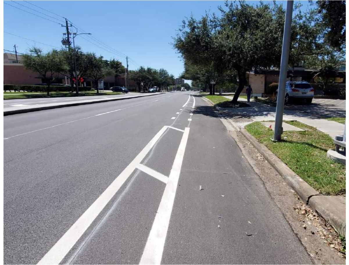
After Construction – Waugh Dr. South of W. Dallas St *
