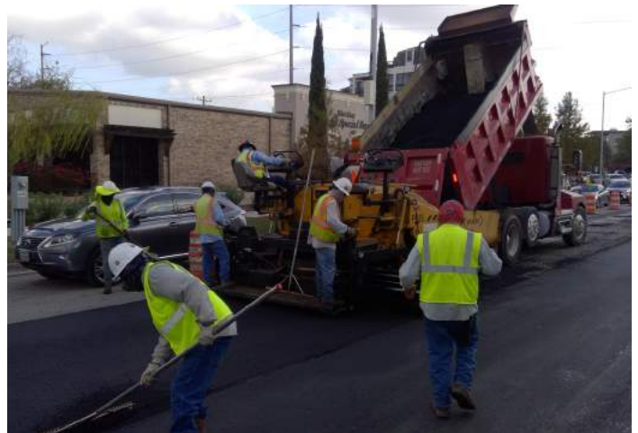
Overlaying Asphalt
