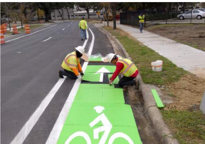
Bicyclist pavement marking installation.
