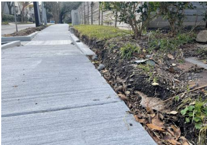
Substantial Completion Walkthrough — Add Retaining Wall
