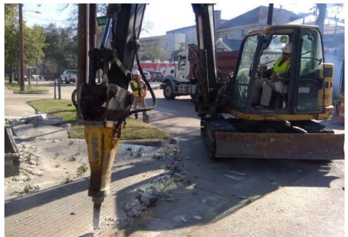
Ramp demolition in progress—Montrose Blvd
