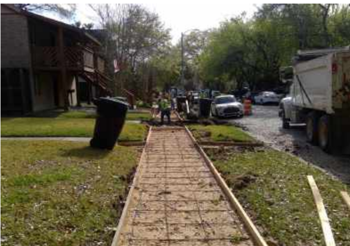
Sidewalk Formwork/Reinforcement Steel Installation
