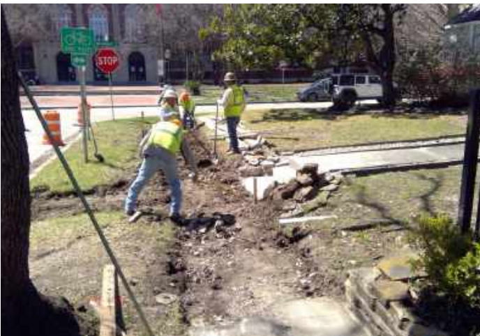
Existing Sidewalk Demolition
