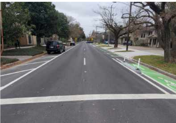
Striping, Signage and Pre-cast Curb Completed.
