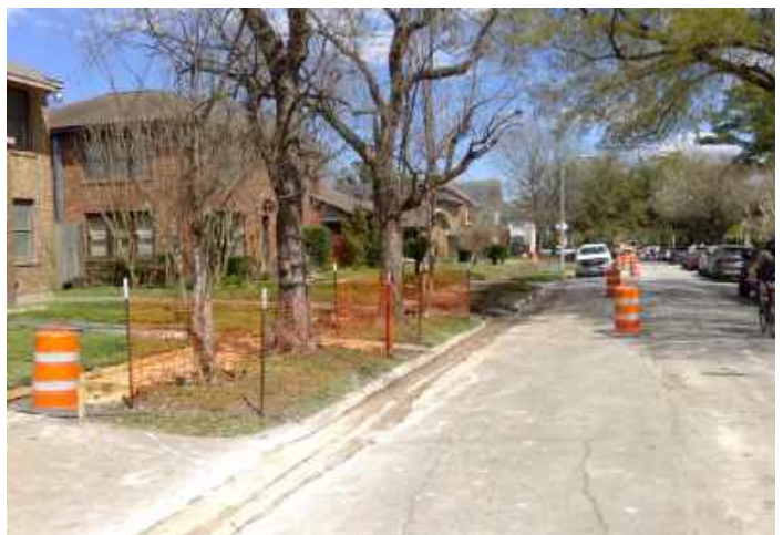
Traffic Control Configuration and Tree Protection
