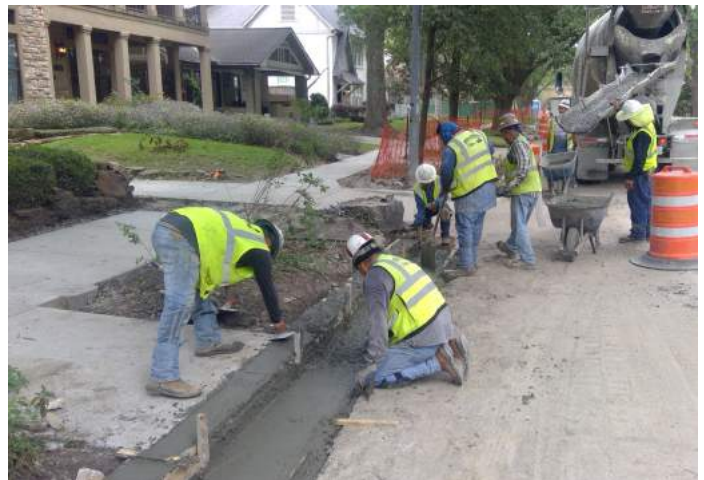
Curb and Gutter Installation
