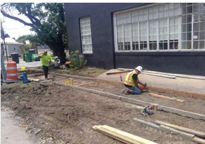
Sidewalk Formwork Installation
