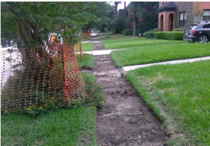
Existing Sidewalk Demolition
