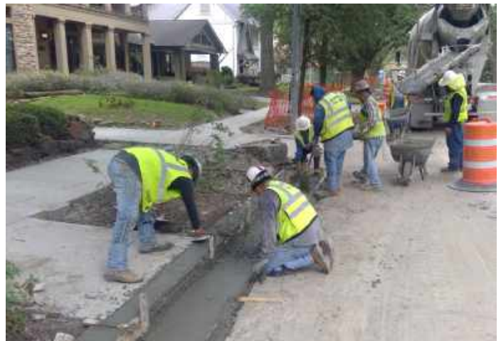
Curb and Gutter Installation
