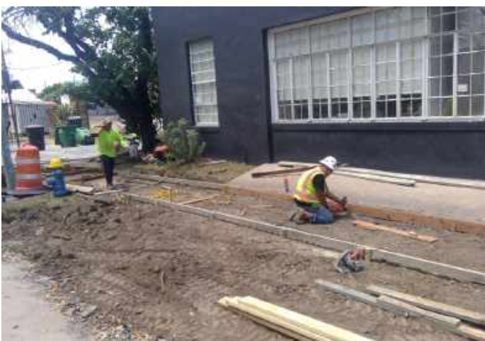
Sidewalk Formwork Installation
