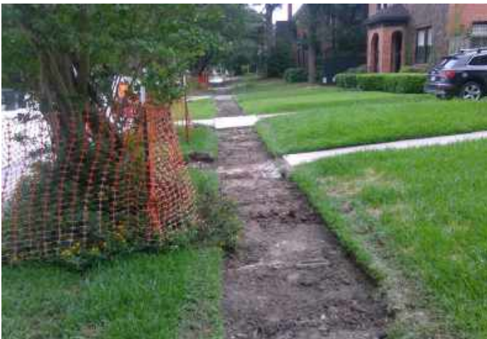
Existing Sidewalk Demolition
