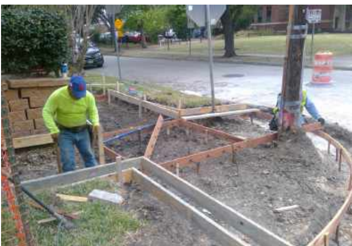
Wheel Chair Ramp Installation
