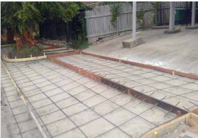
Driveway Formwork
