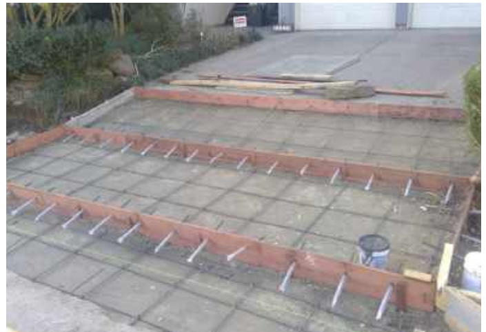
Forming work for Sidewalk and Driveway
