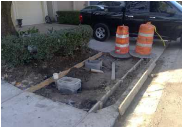
Remove & Replace Water Meter Box
