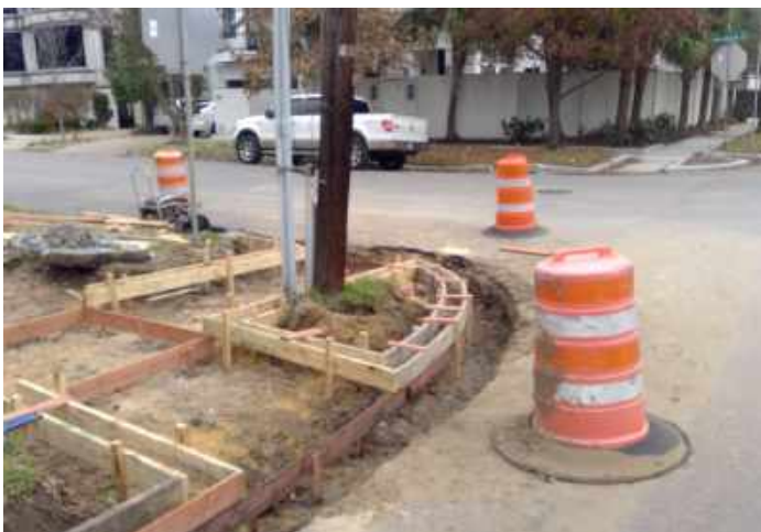
Forming work for Curb Ramp
