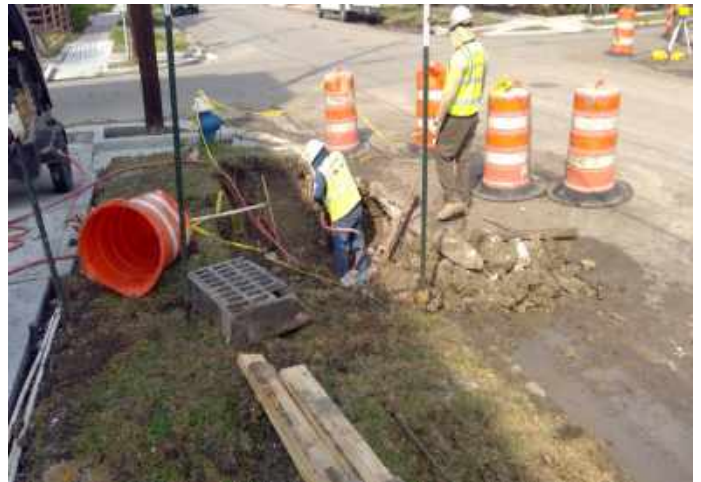
Replacing old Inlet
