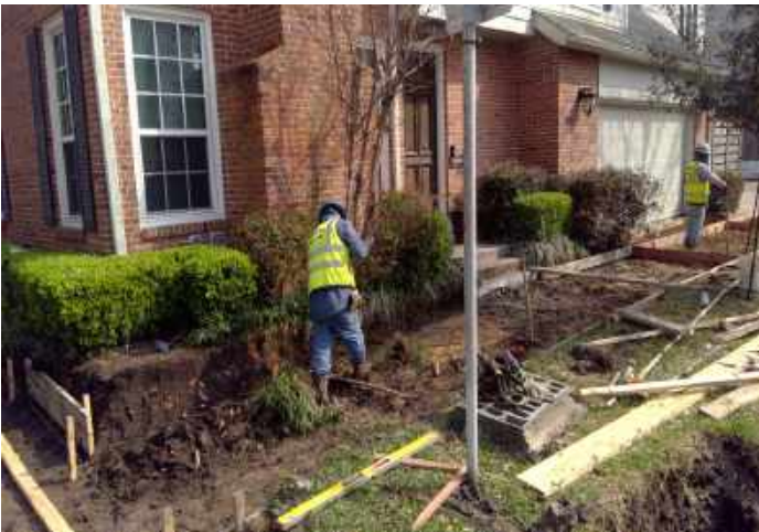
Forming work for Sidewalk
