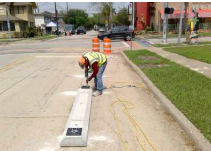
Bike Lane Precast Curb and Bollard Installation
