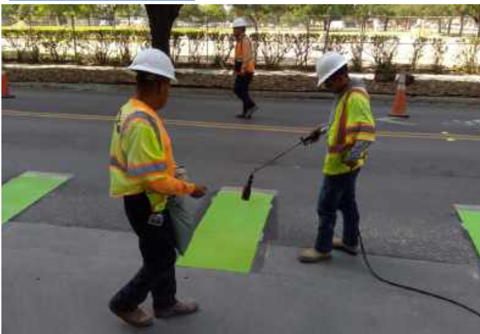
Bike Lane Striping
