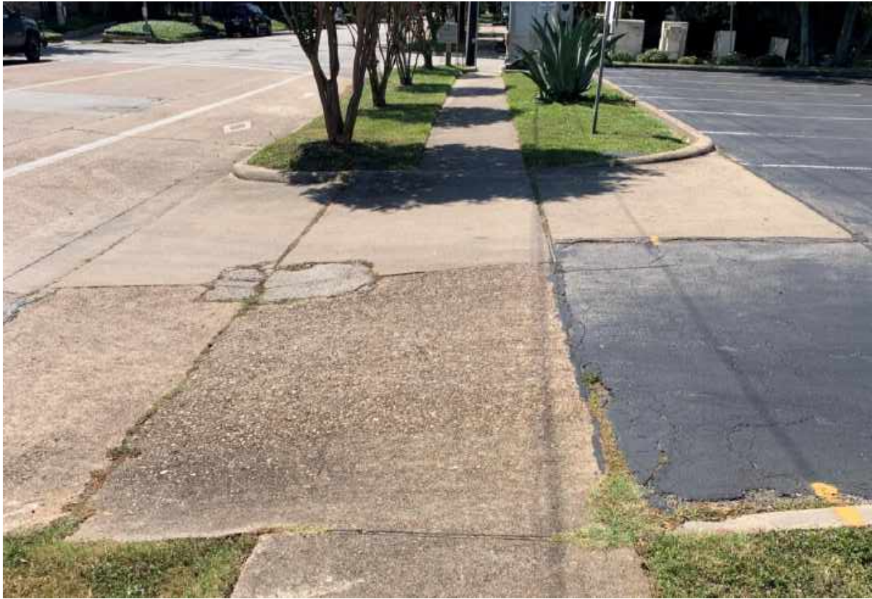
Before Construction Commonwealth St South of Vermont St
