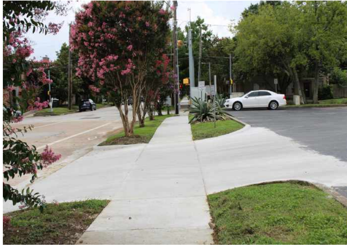
After Construction Commonwealth St South of Vermont St
