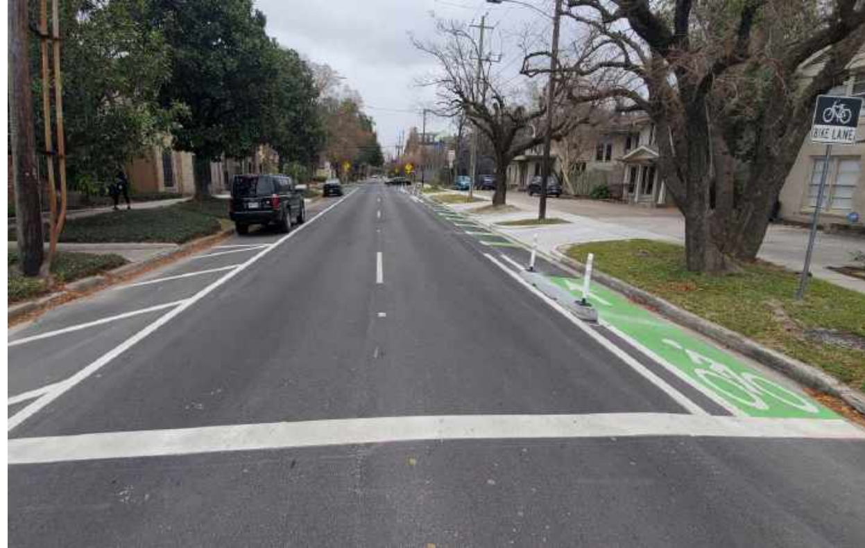
After Construction Commonwealth. South of Welch St
