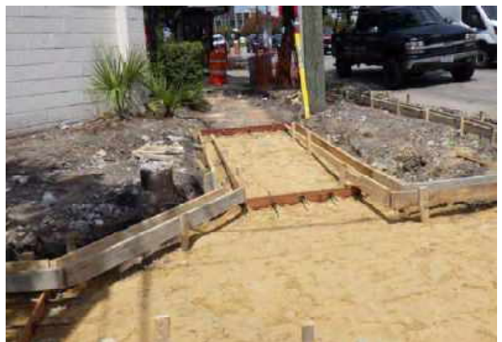
Ramp Formwork Installation
