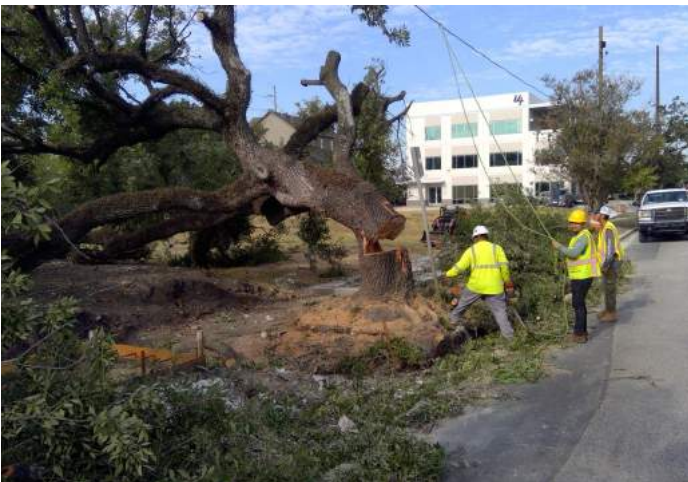
Dieback Tree Removal
