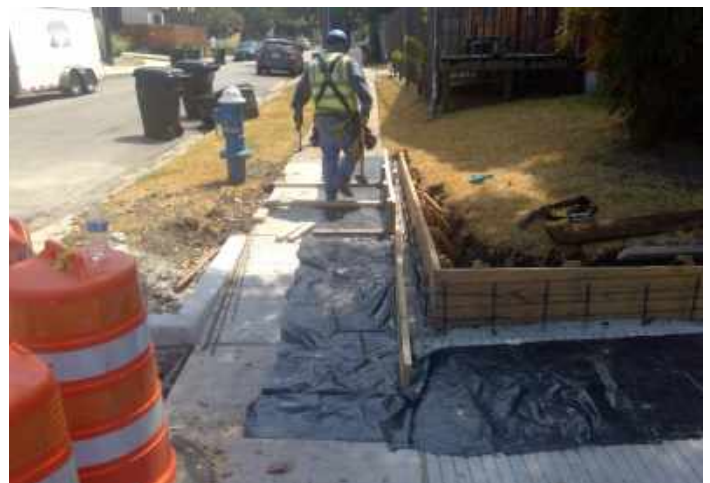
Curb Wall Form Work
