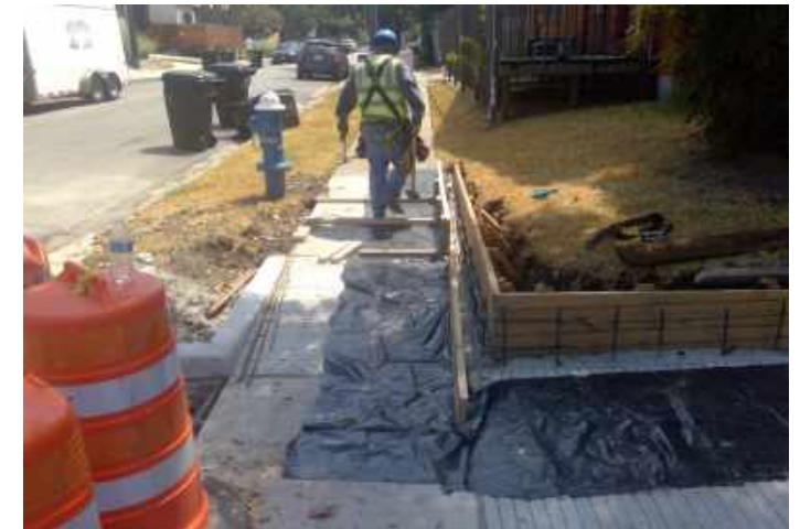
Curb Wall Form Work
