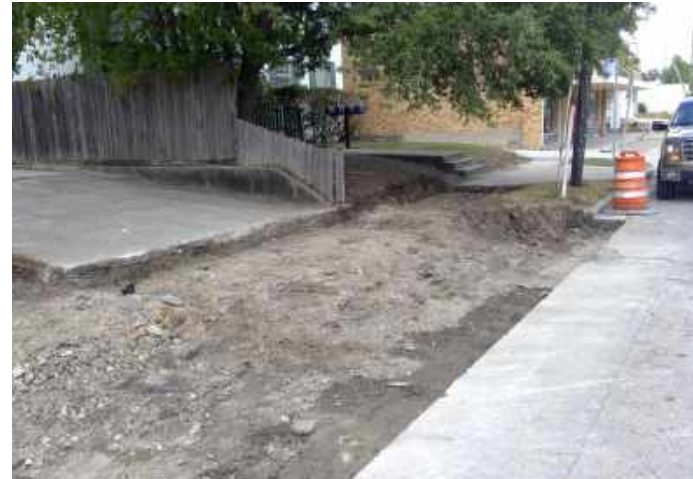
Concrete Removal
