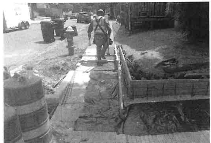
Curb Wall Form Work
