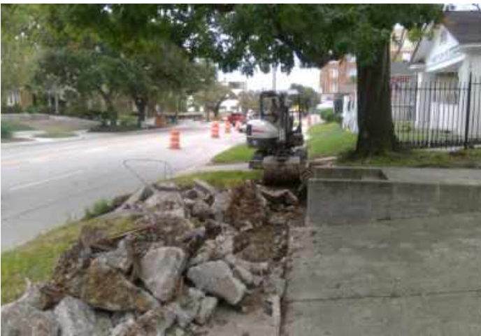
Removal of Existing Concrete
