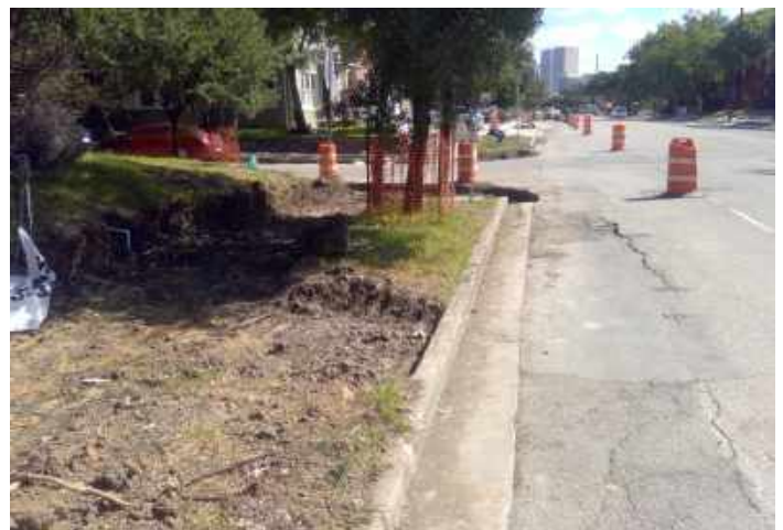
Traffic Control/Tree Protection
