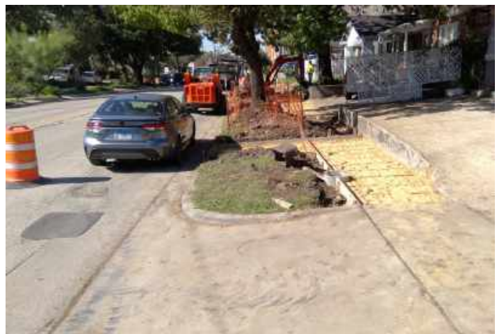
Traffic Control/Tree Protection
