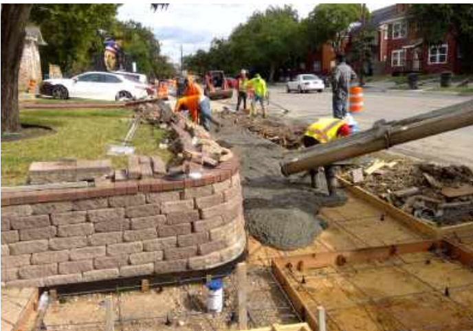
Pouring Concrete for Sidewalk
