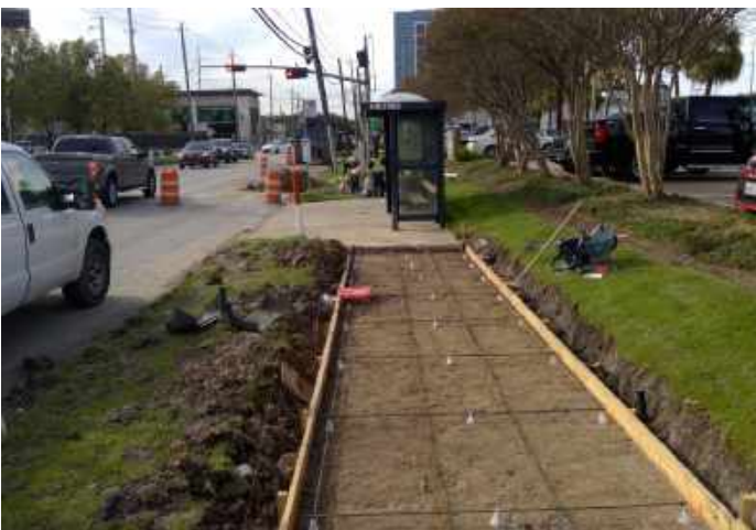
Formwork Installation for Sidewalk
