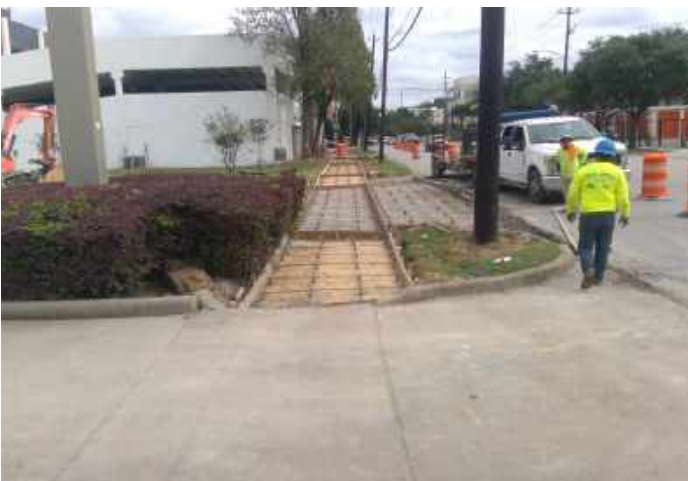
Formwork Installation for Sidewalk
