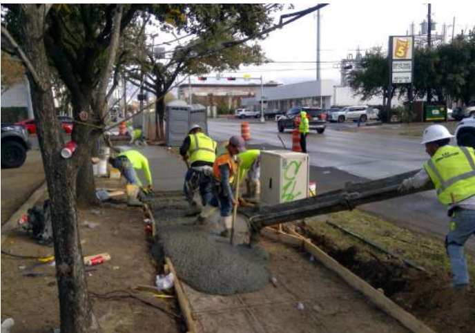
Pouring Concrete for Sidewalk
