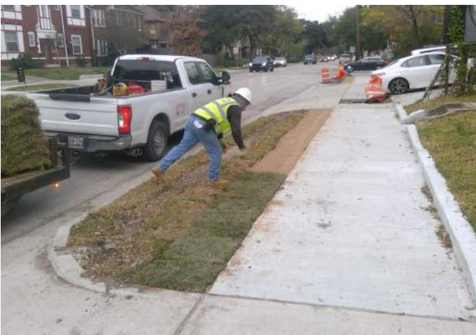
Placement of Coarse Sand/Sod
