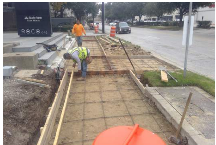
Installation of formwork for bus pad replacement
