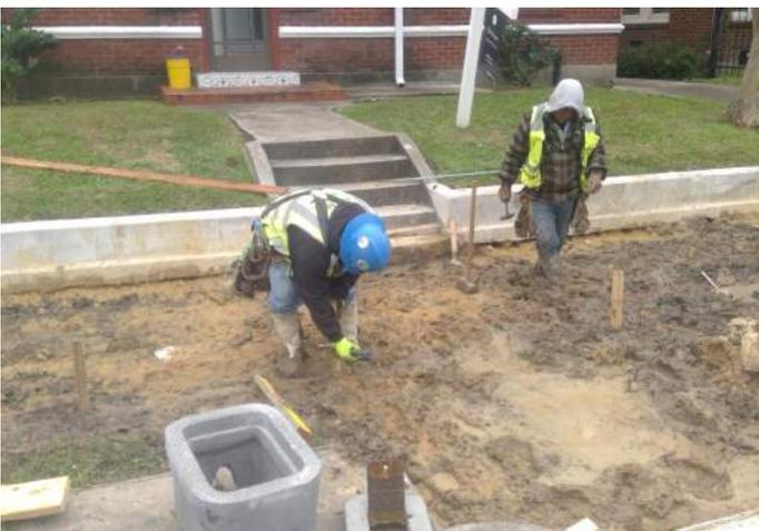
Reconstruction of Sidewalks of Non-compliant Cross Slope
