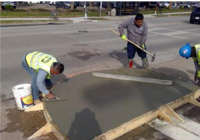
Pouring Concrete for Median Nose
