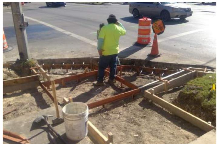
Installation of Formwork for Curb Ramp Replacement
