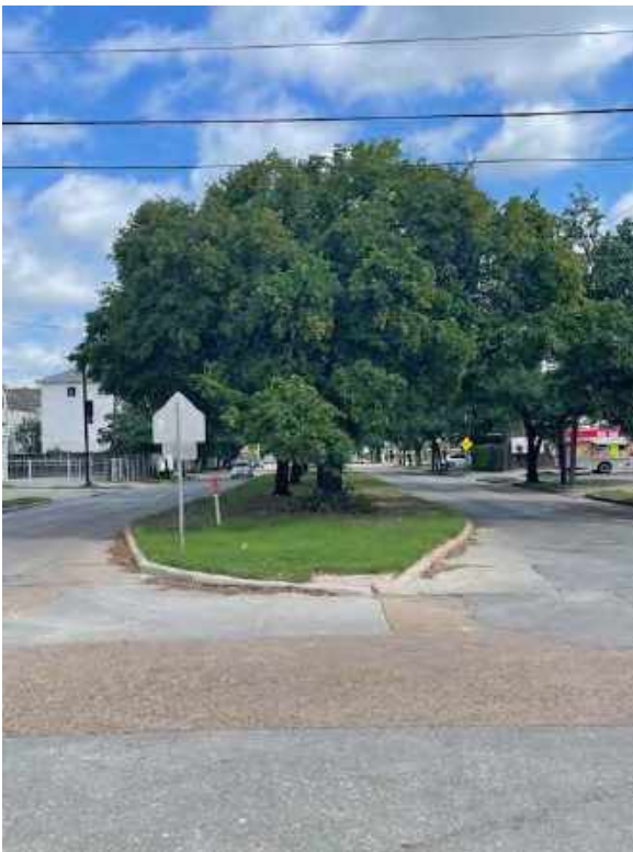
Phase One median trees planted in the center to avoid impacts if the 1970s plan to add a third lane in each direction was implemented. The roadways now will be shifted into the median about half of the originally planned distance.
