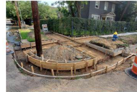
Ramp framework installation
