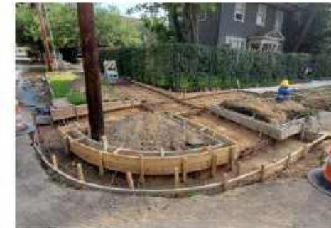
Ramp framework installation
