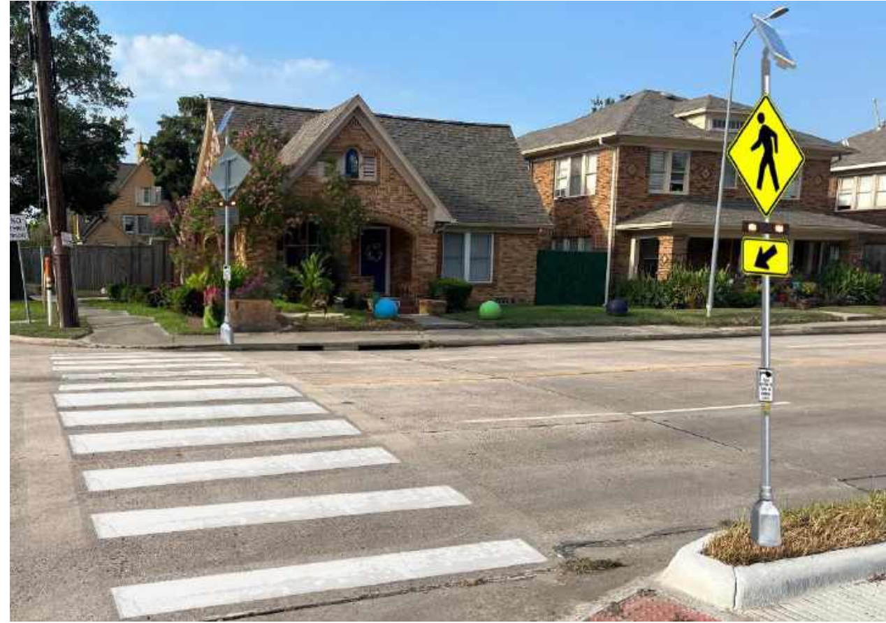
Rectangular Rapid Flashing Beacon at Stanford at W Dallas
