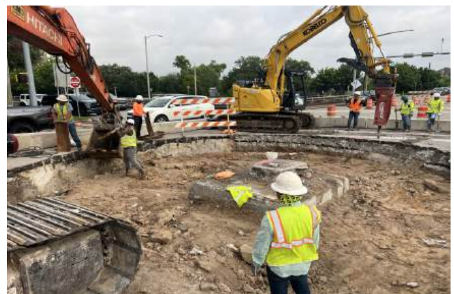
Excavation for Junction Box Installation
