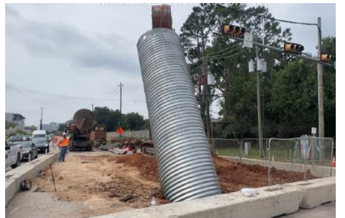
Temporary Manhole Installation
