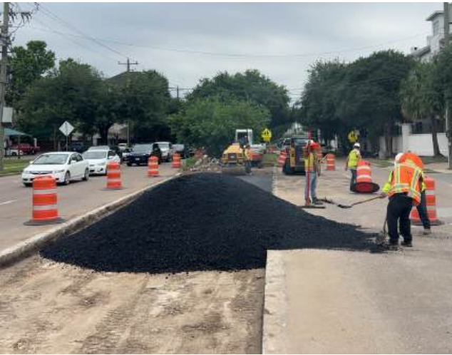
Temporary Asphalt Installation
