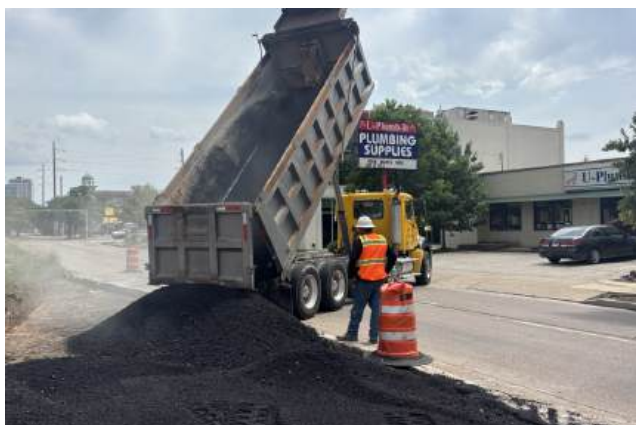
Temporary Asphalt
