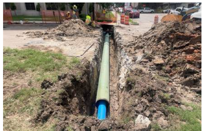
Water Line Installation
