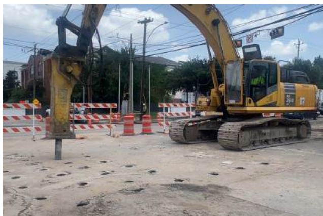
Intersection Pavement Removal
