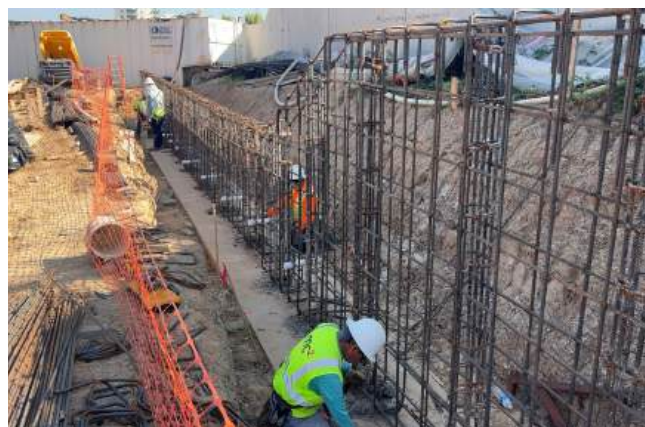
Retaining Wall Installation
