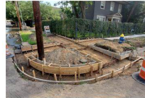
Ramp framework installation
