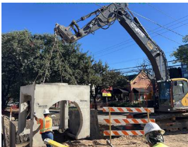
Storm Structure Installation
