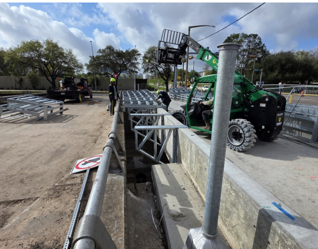
Cladding System Supports
