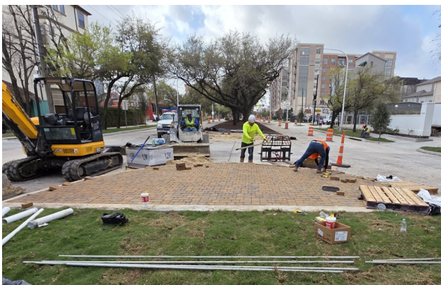
Pavers in Median
