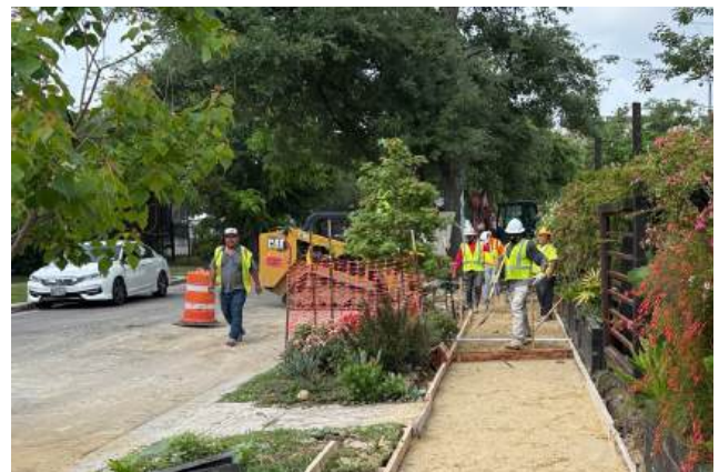
Tree Protection Fencing
