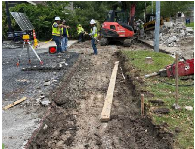
Sidewalk and Driveway Demolition
