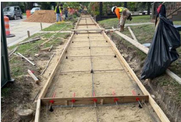
Sidewalk Formwork
