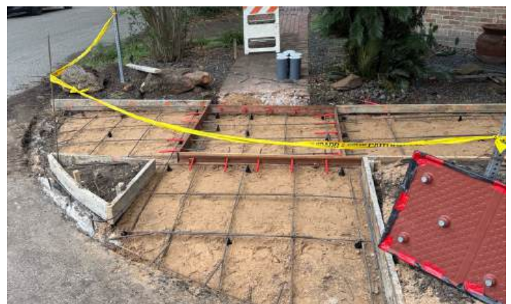
Sidewalk Ramp Improvements
