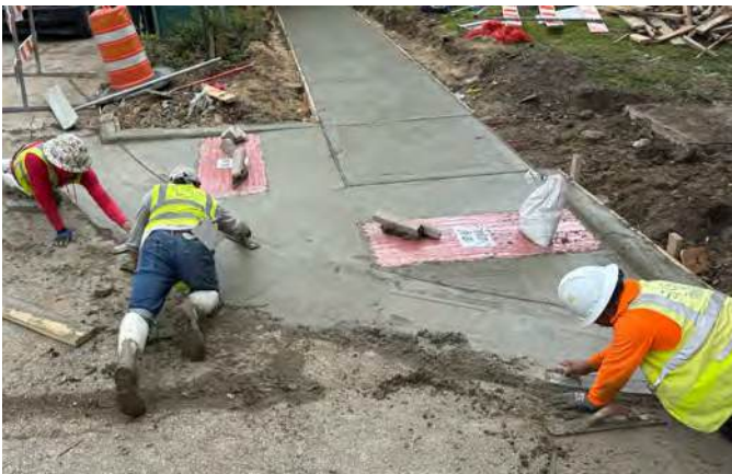
ADA Ramp Improvements
