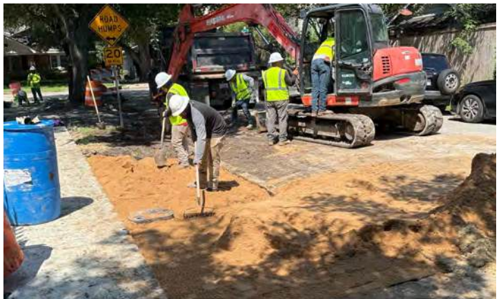
Haver St. Parkway Restoration
