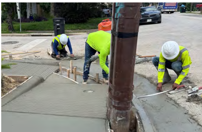
ADA Ramp Improvements
