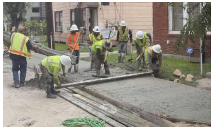
Placing Concrete Sidewalk
