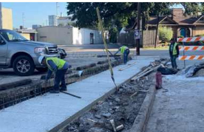
Curb Wall Reinforcement
