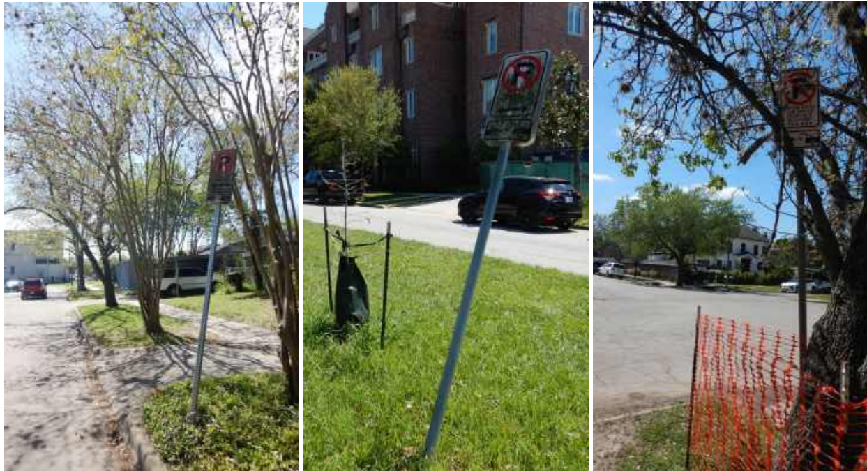
Figure 52. Faded and hard to read signage across the study area
